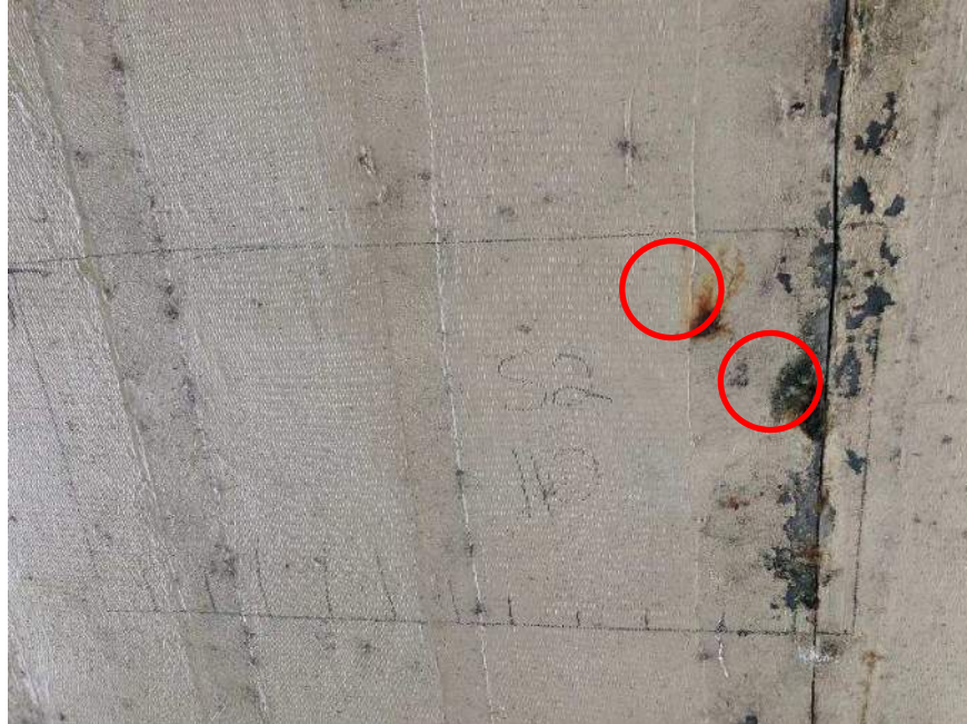
Rust staining and active seep, downstream center of Span B
