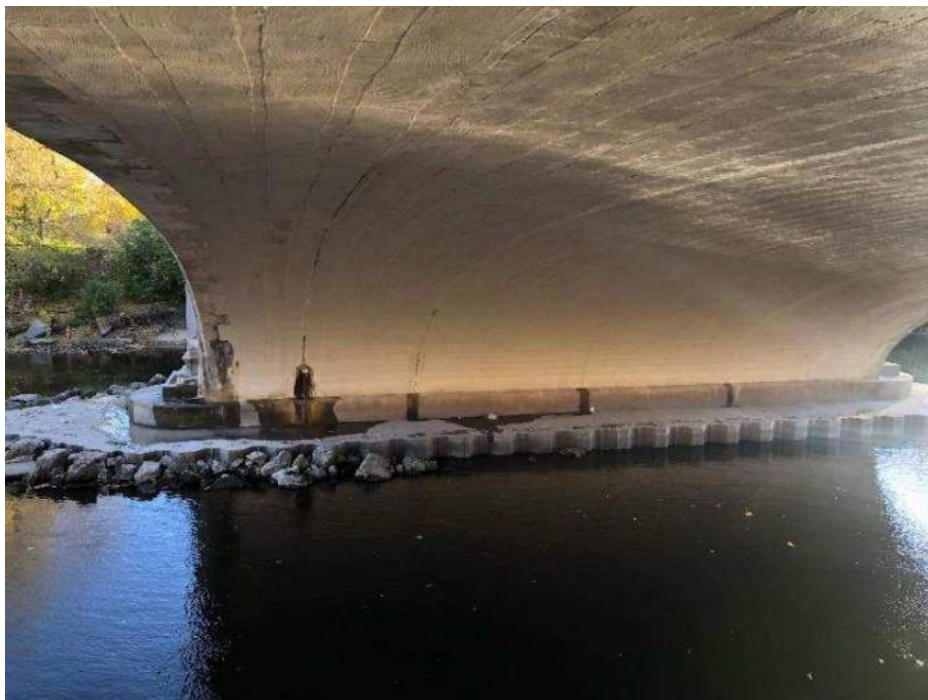
The north side of Pier 2 while performing Test Core TC-2. Water exiting the drain, arch joints and façade.
