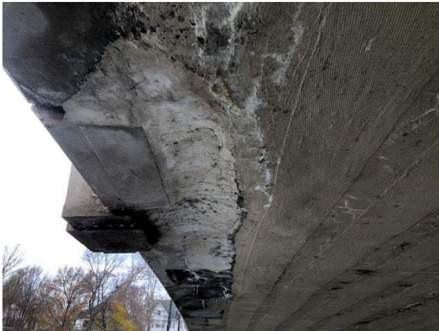
Mineral crystallization, downstream center of Span B
