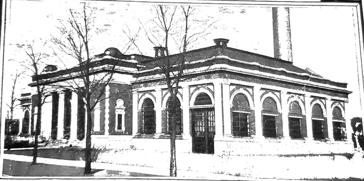
North Pumping Station — Completed 1914
